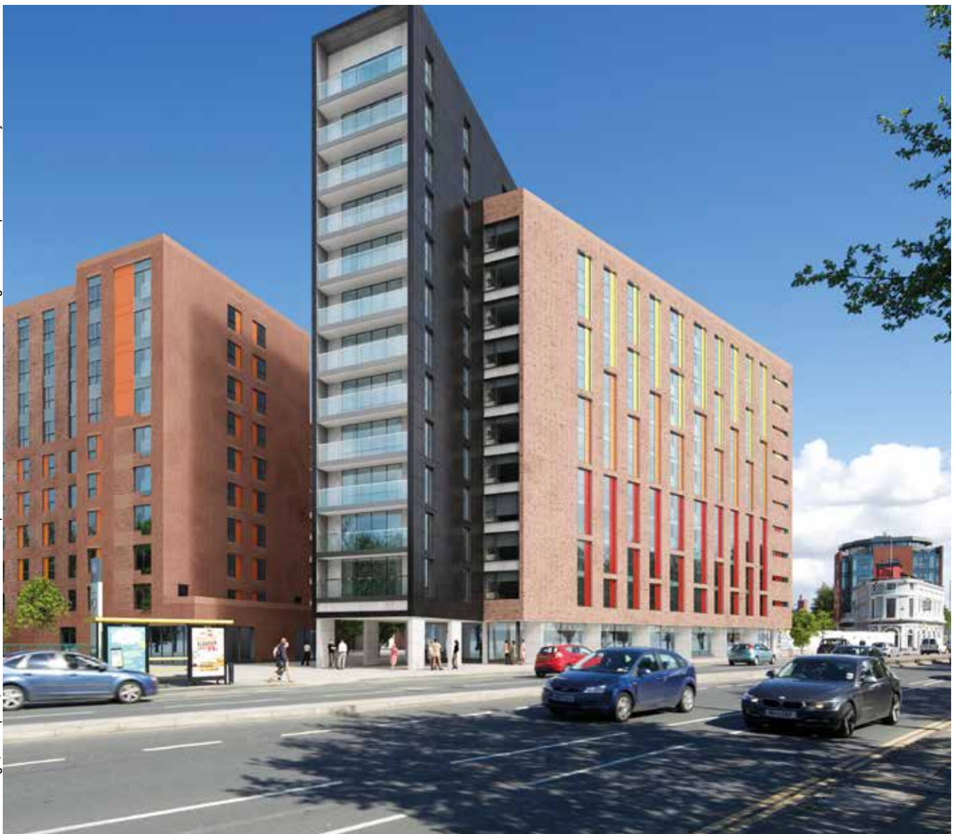
Baltic Village, Liverpool, 324 Private Rented Sector Apartments & communal facilities - Image of Development underway
